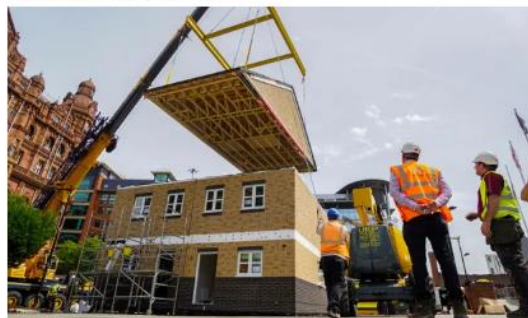
▲ The like homes are bolted together on site, with the record for assembling a property standing at 36 hours. Photograph: Ilke Homes
